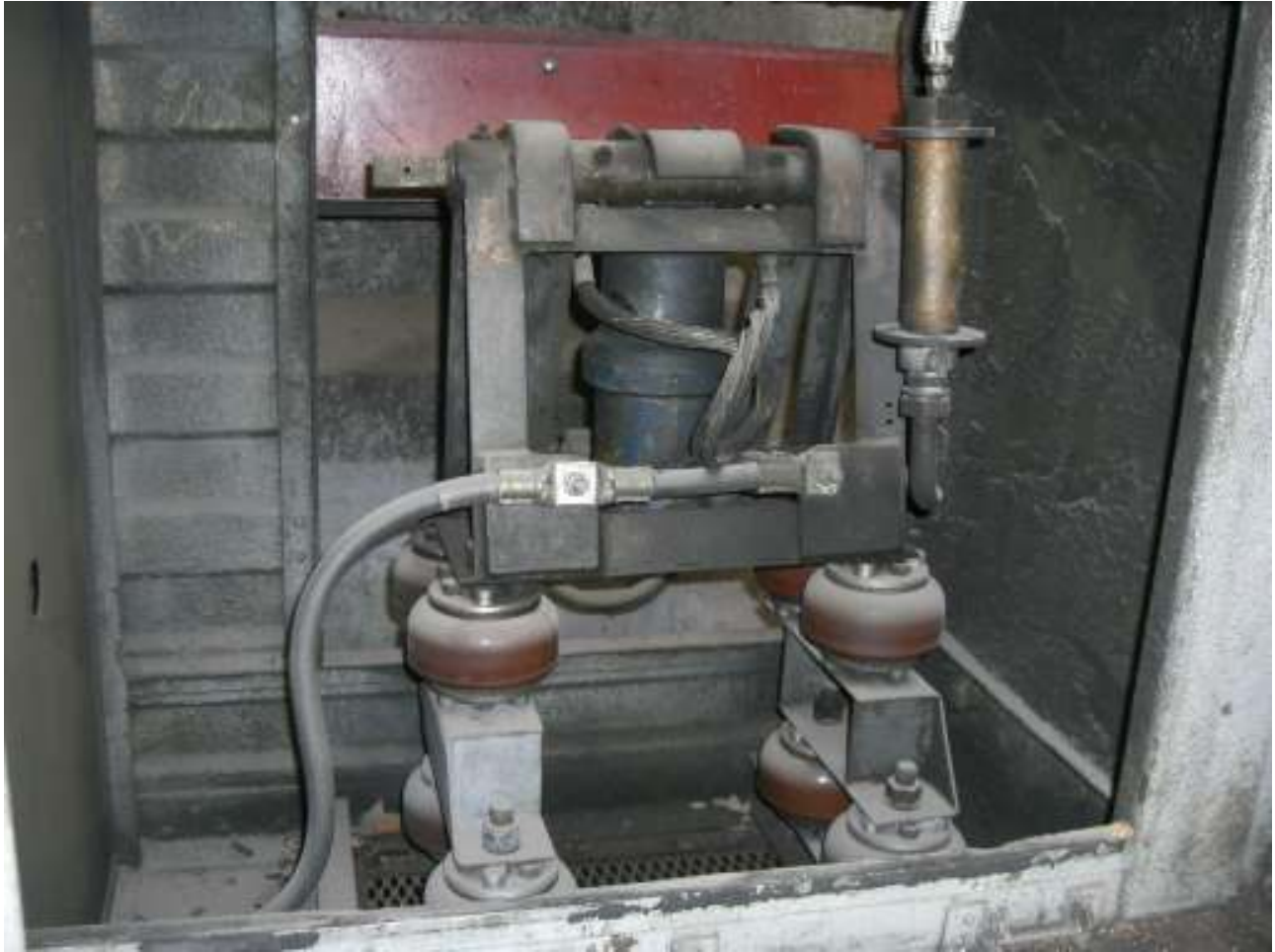
Positive Collector Assembly shown installed in collector compartment
