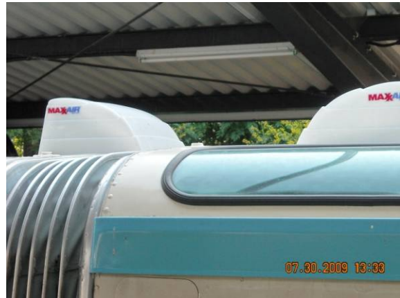
Install new roof vents and seal the edges to prevent leaking.
